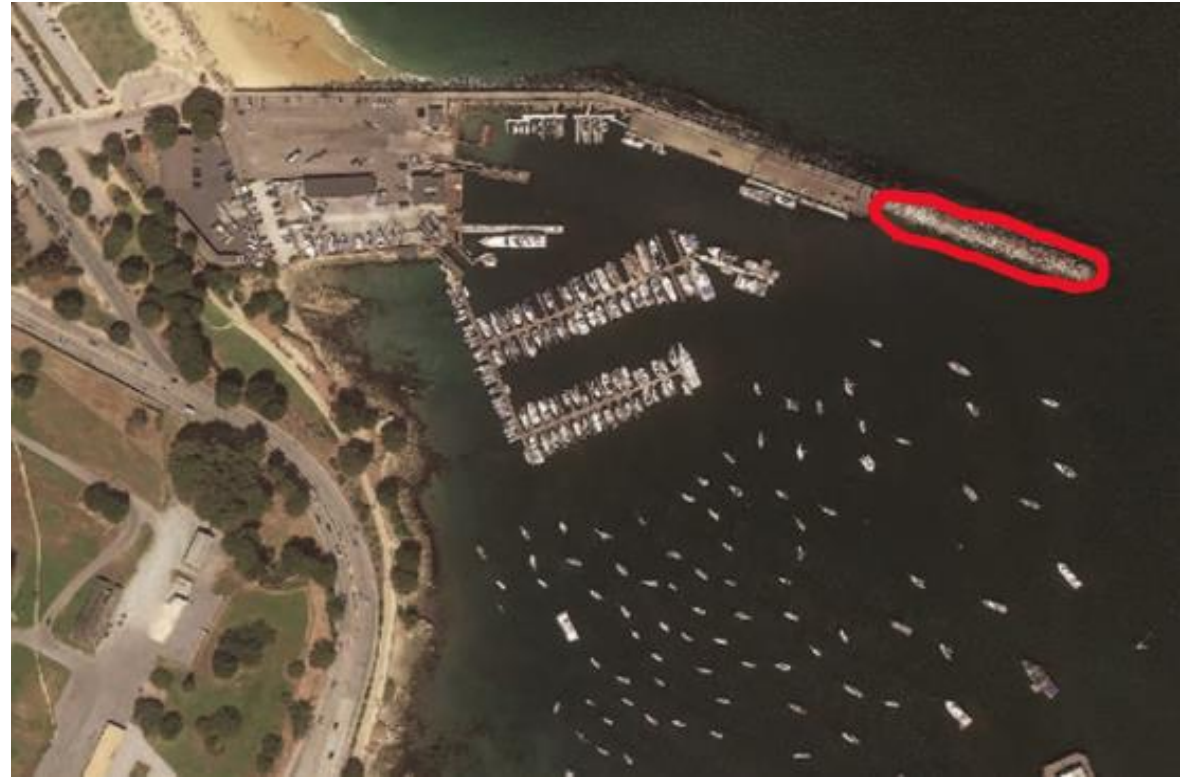
Monterey Coast Guard Pier
